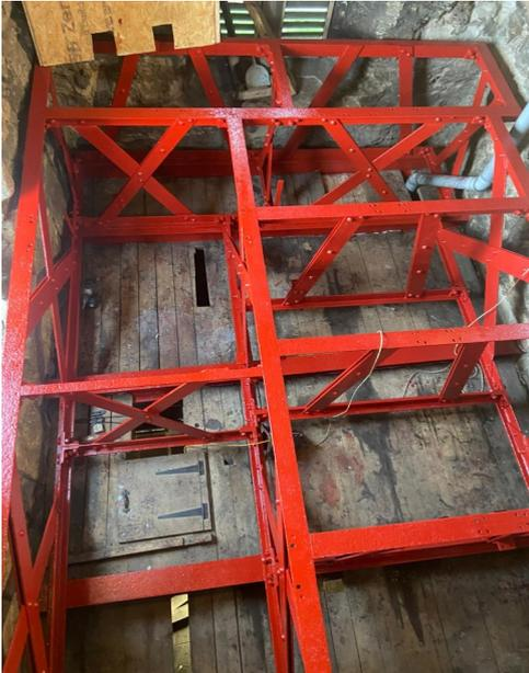
Early in September two contractors, employed by Taylor's, removed as much of the dirt and corrosion from the bell frame and painted on some rust inhibitor. That took a couple of weeks to seep into the metal and dry. Then, in the week of 20<sup>th</sup> September they returned and helped by Rohan Wanduragala, Thelma Adams and Andrew Frost, they applied zinc primer and then a red enamel top coat to the frame. The image shows the frame ready to receive the bells.
